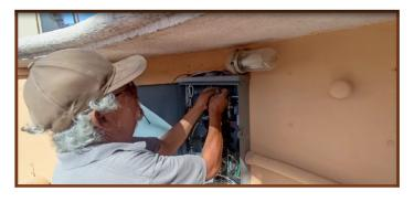
The wiring was also replaced and a new electrical box was installed.
